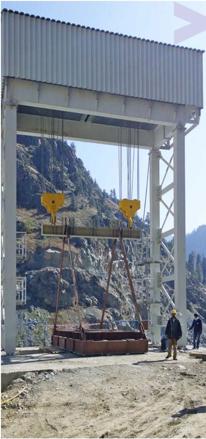
The protective enclosure of the hoisting technology from STAHL CraneSystems was manufactured by its certified partner Haslinger GmbH Metallbau + Krantechnik.
